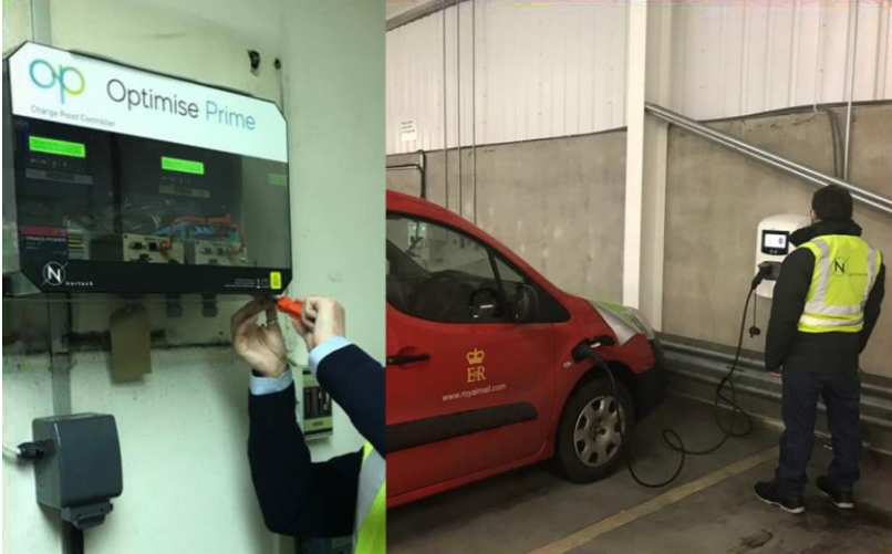
Figure 4 – Installation and testing of CPC infrastructure. Images courtesy of Nortech.
