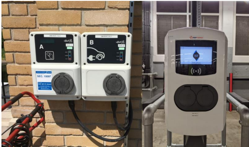
Figure 5 – Legacy Swarco eVOLT twin (left) and newly installed Alfen twin (right) CPs at Royal Mail Depots
